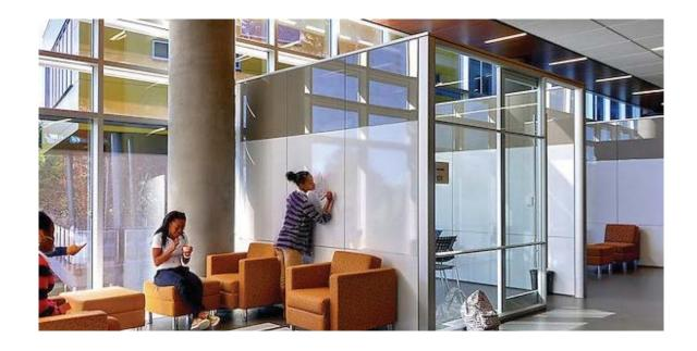
Easy to configure (demountable) interior wall systems will be employed where program requirements define and support the need for functional change and flexibility.
