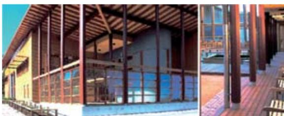
**Figure 38:** (Left) Two-story wood building with simple roof forms but sufficient detailing of fence, shading devices and long eaves to provide visual richness; (Right) Large canopies between the inside and outside increases the spatial experience and allow children to play safely on all sides of the building. (Hosmarinpuisto School and Day Care Centre, Espoo, Finland – Illustrative Case)
