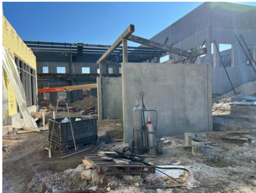
Exterior kiln walls stood into place
