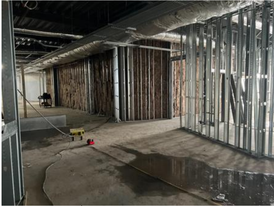
Drywall and insulation 2 nd and 3 rd floor
