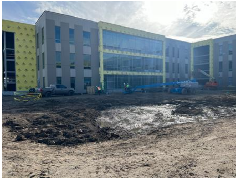
Curtain wall glass installation
