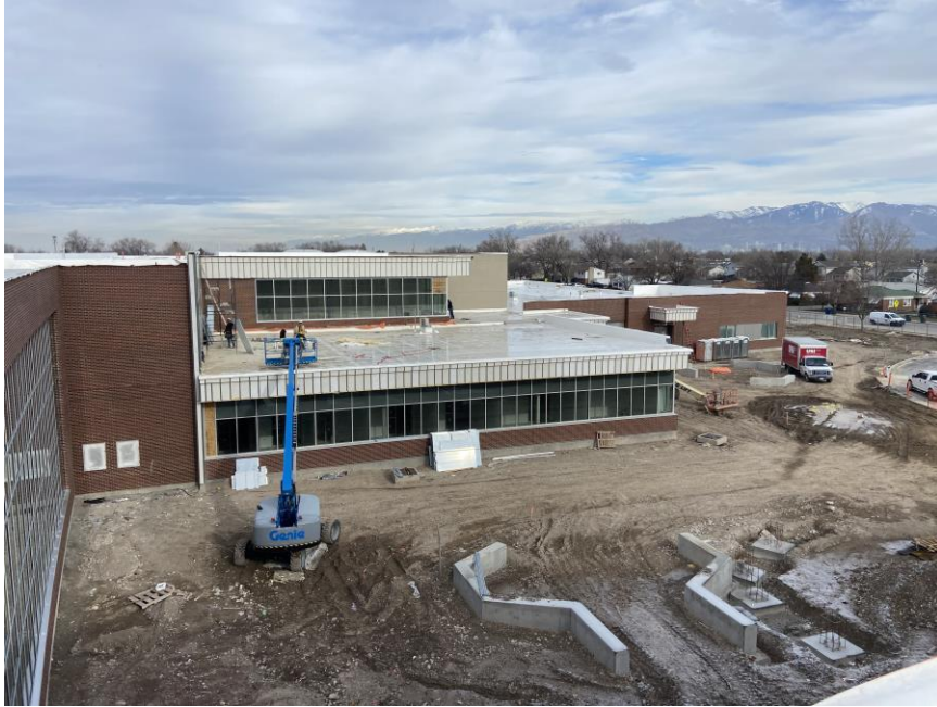
Insulation and decorative metal panels
