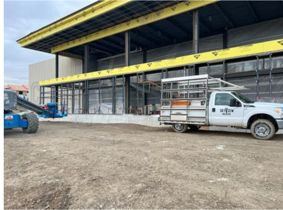
Vestibule curtain wall installation
