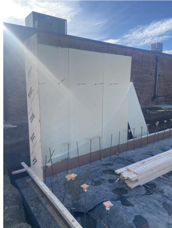
Concrete forms for walls
