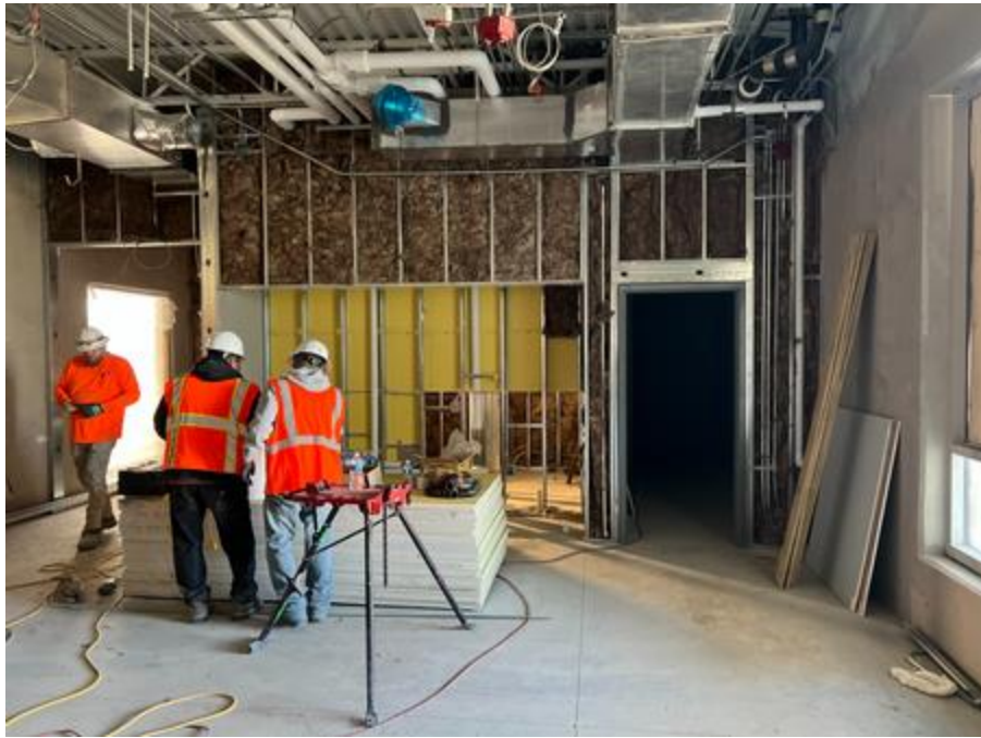
Locker room framing, drywall, and plumbing
