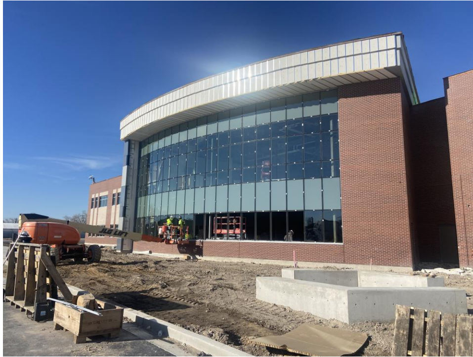
Glass installation at building exterior
