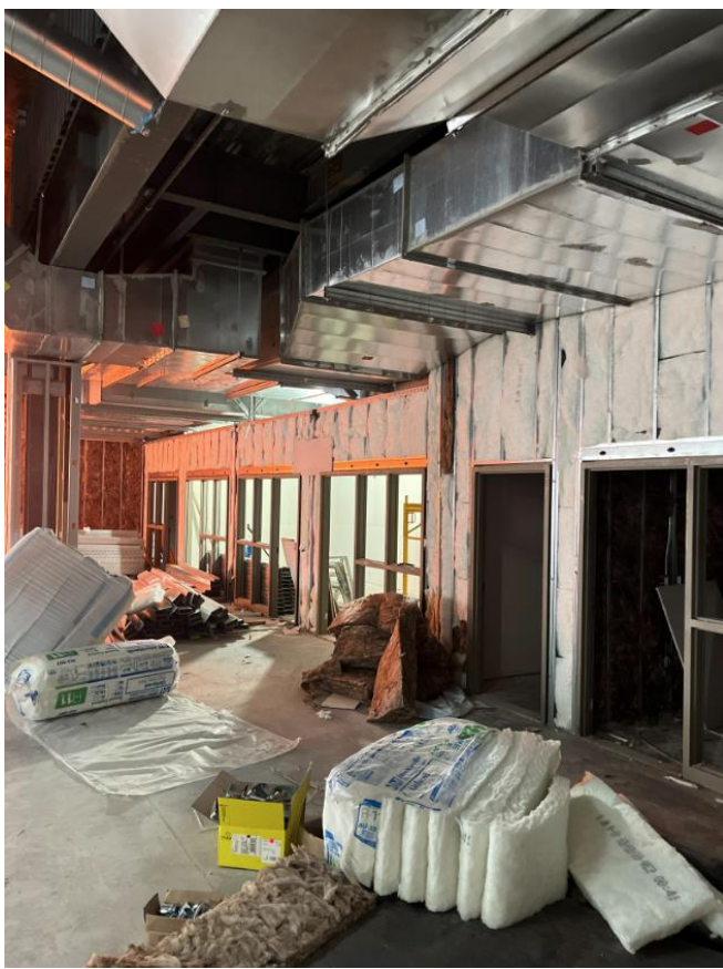
Media Center walls insulated, ready for sheetrock
